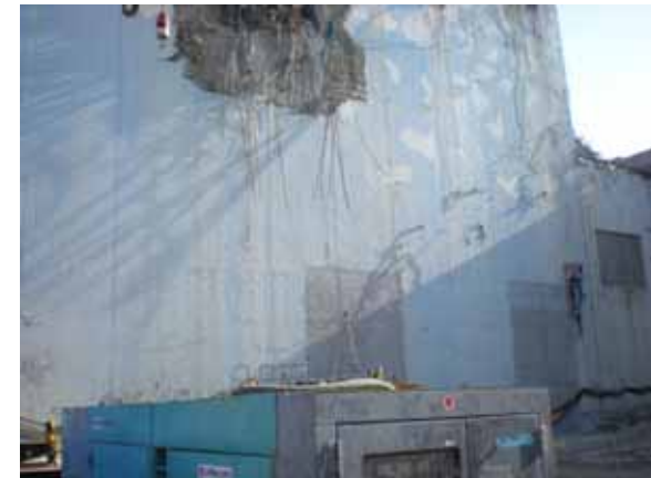
⑥ South wall (Exterior wall)
