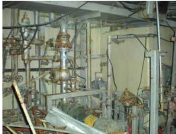
⑦ Wall on the SFP side (West)
