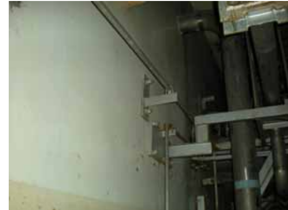
⑧ Wall on the SFP side (South)
