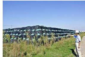
Sludge containing radioactive cesium. Covered with black liner sheet, are stored in the outdoors (15 days, in the purification plant Okubo, Saitama)
