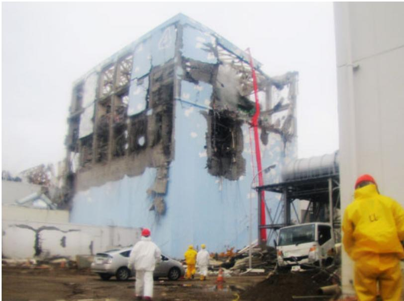
Pump it up: Water-spraying operations to cool down a spent nuclear-fuel pool at the Fukushima No. 1 power plant's No. 4 reactor continue Tuesday with trucks using a concrete squeeze pump and a 50-meter arm for pouring water from a higher point. KYODO PHOTO
